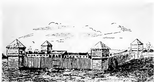
A PALISADED FORT
